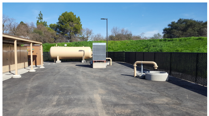
ARC Water Well Replacement
