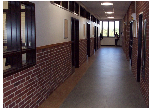
SCC Rodda Hall North 3rd Floor Remodel
