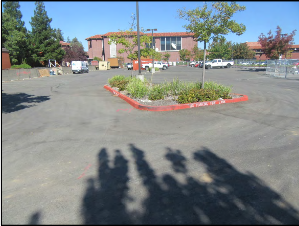
Parking lot "F", east of Mohr Hall and Lillard Hall, looking northeast from near Sutterville Road; 10/16/18.
