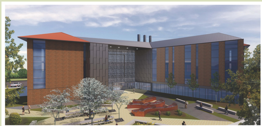
SCC Lillard Hall Science Building
