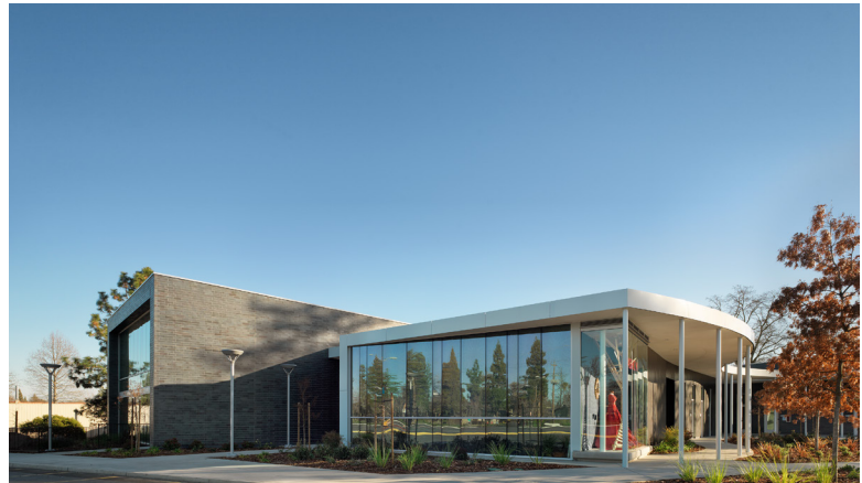
ARC Life Science & Fine Arts Modernization
