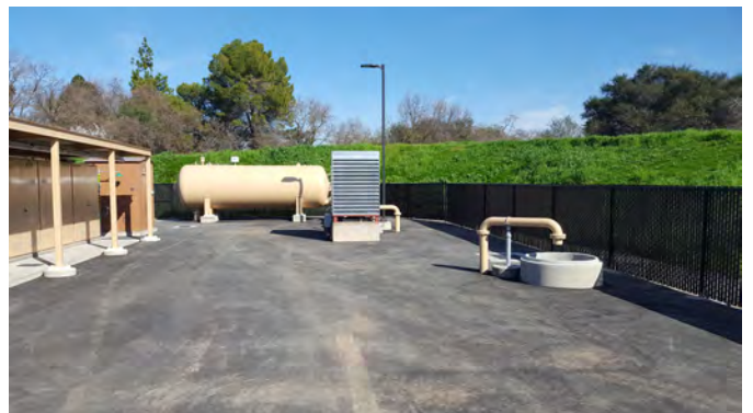
ARC Water Well Replacement
