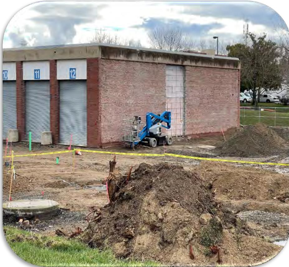
Selective Demolition of Brick at North Wall complete and Site Subgrade in Progress
