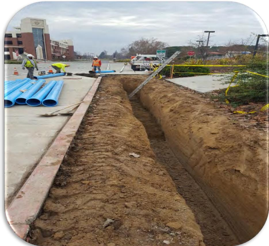
Site Utilities - Fire Water Line Installation – final connection will complete the Loop and provide optimum fire water delivery
