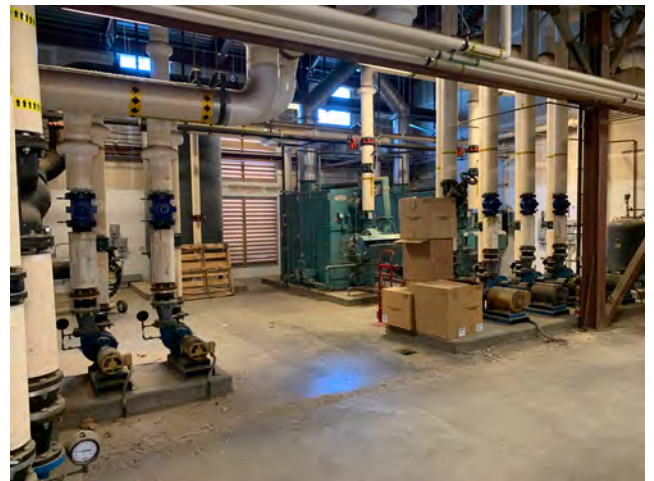
FLC Central Plant Upgrade
