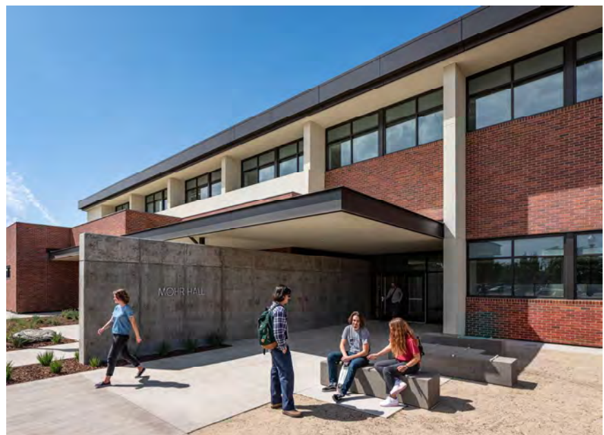
SCC Mohr Hall
