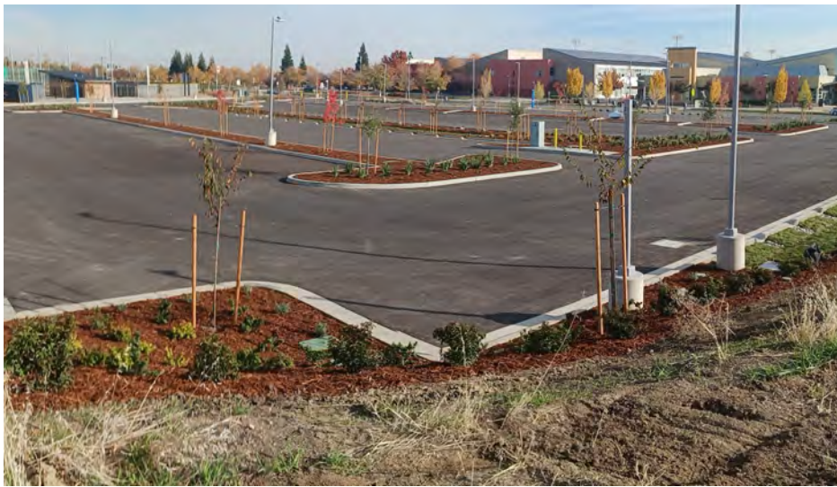
Paving and Landscaping completed looking towards Library
