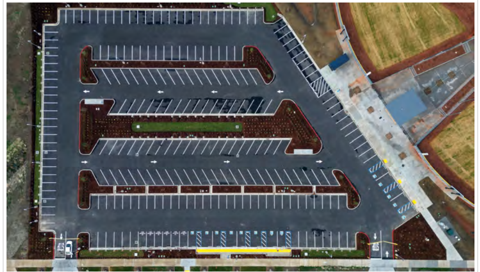
Aerial View of Completed Lot
