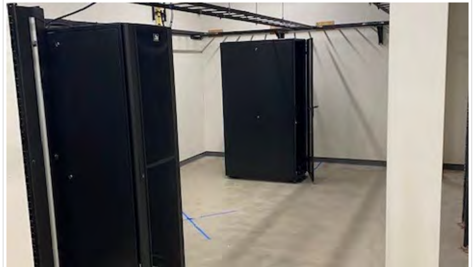
Existing MDF from south
