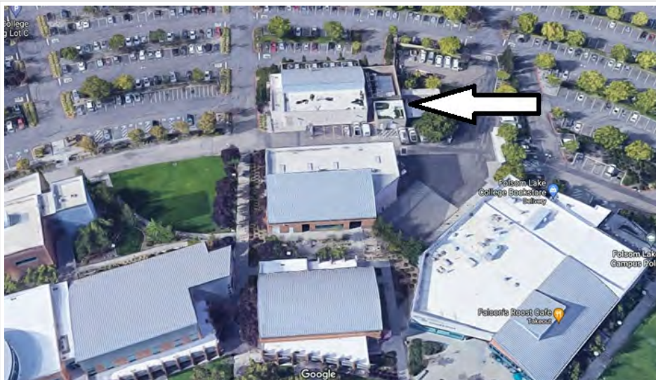
FLC Central Plant
