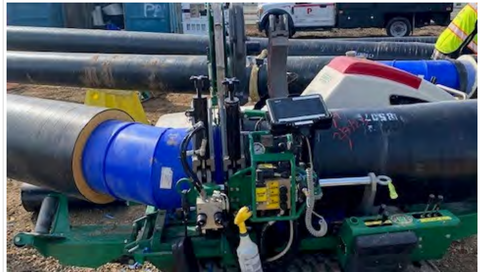
Heat Fusing Hydronic Pipe
