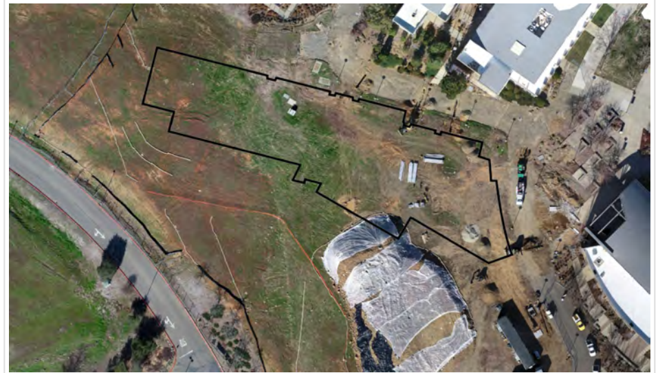
Jan 31 Drone View of Project site
