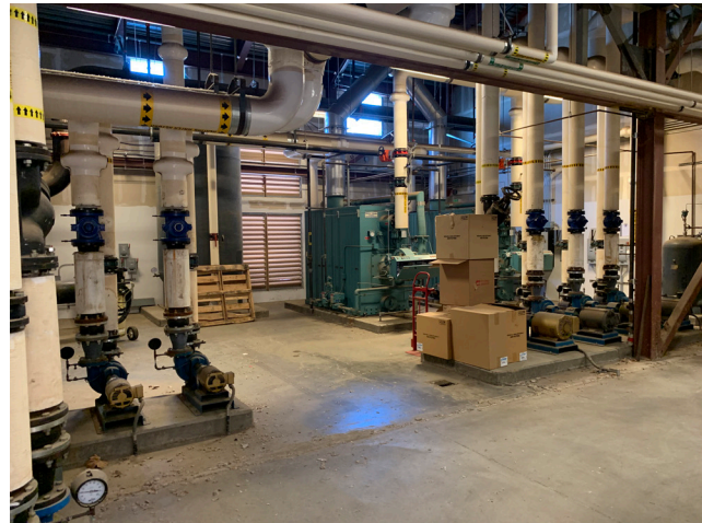
FLC Central Plant Upgrade
