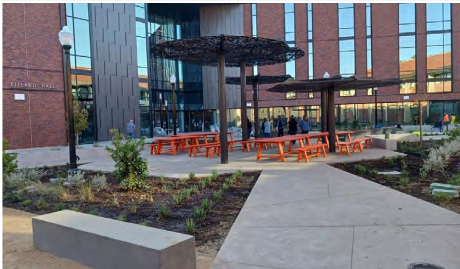
Courtyard West and North Elevation
