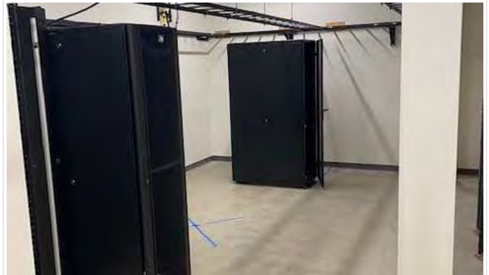
Existing MDF from south
