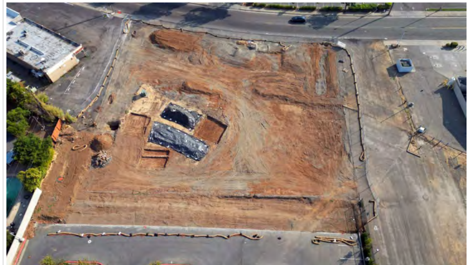
Contaminated Soils Removal Complete
