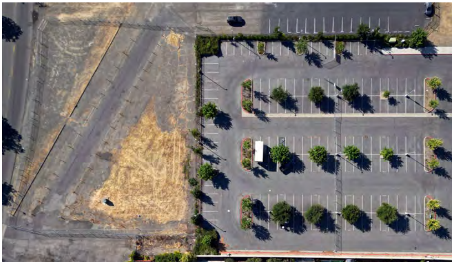
Rancho Cordova Center Parking Lot Extension to Dawes Street Limits
