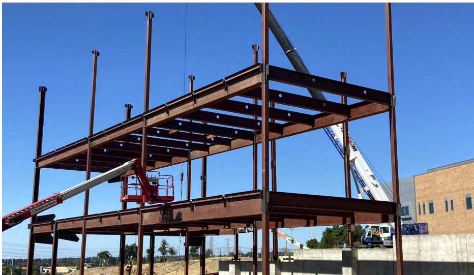
Steel erection progress 10/11/23
