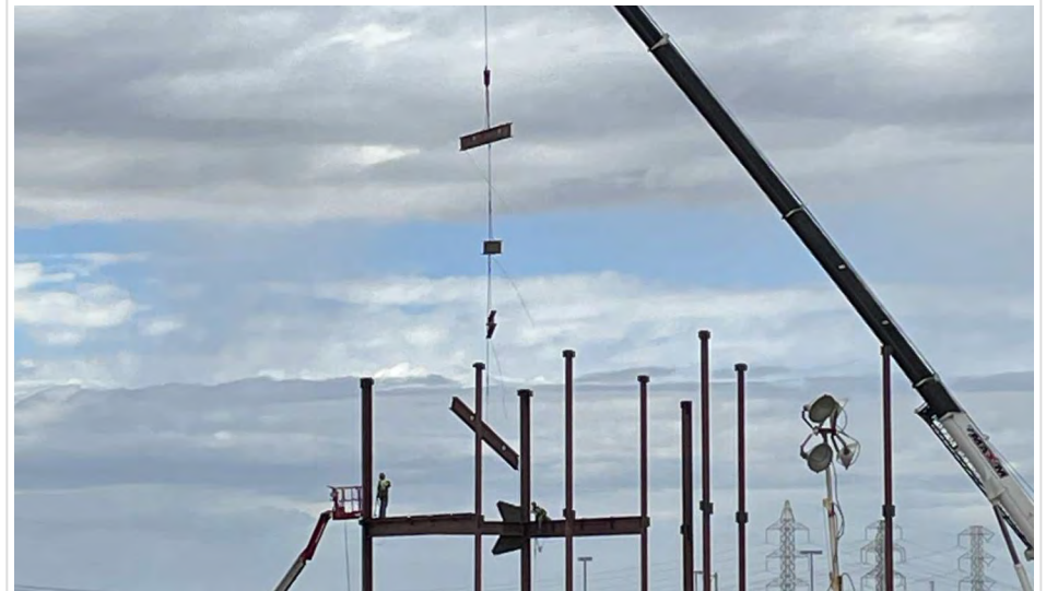
Placement of steel beams
