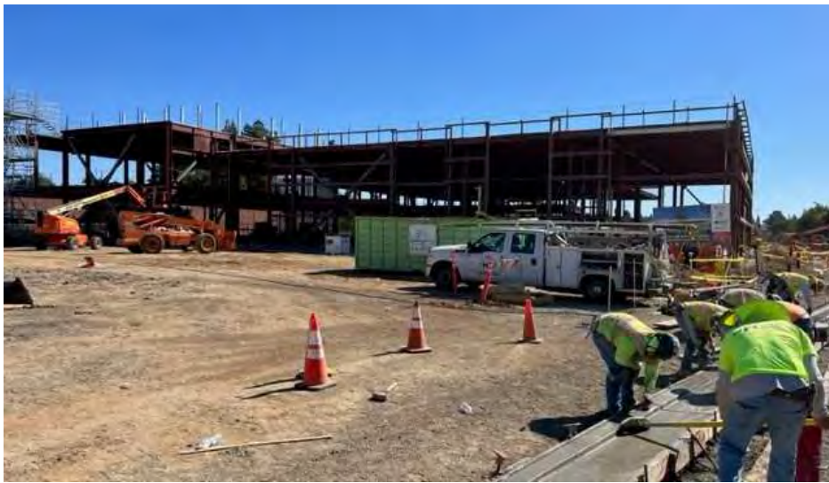
View From North
