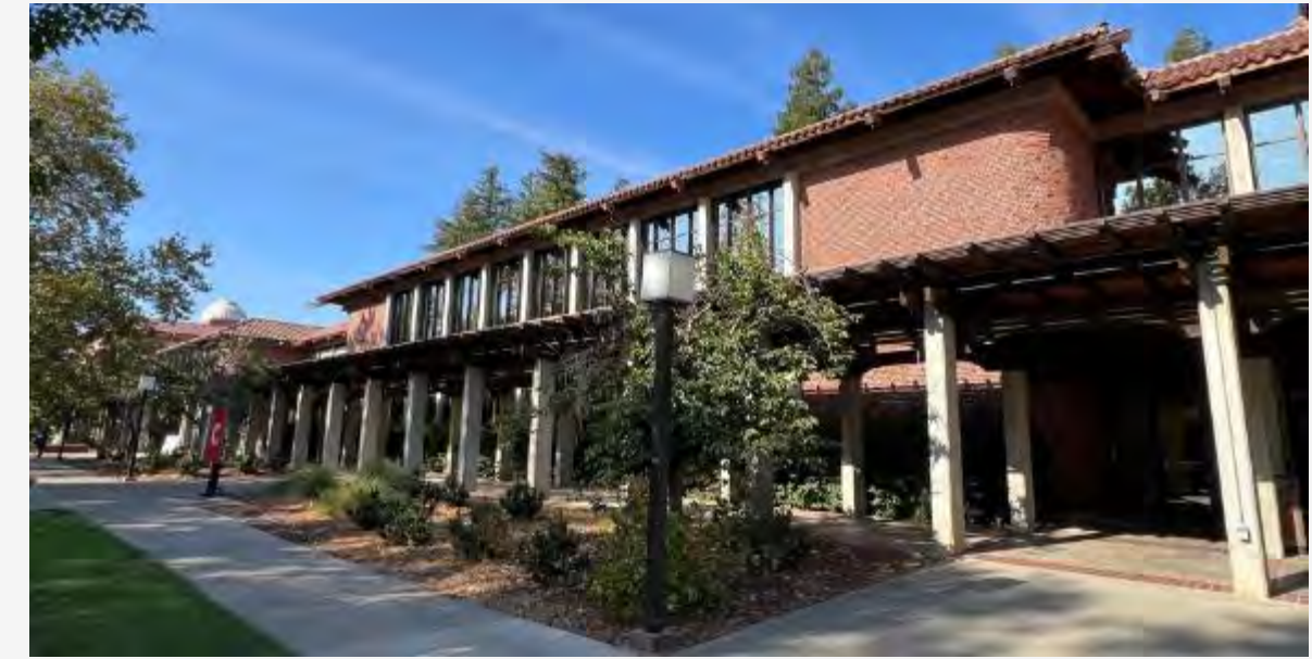
Photograph of Rodda Hall North and South historic architecture
