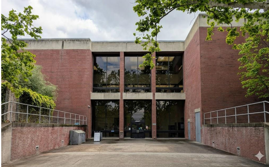
Photo C1 – North Library Entrance
