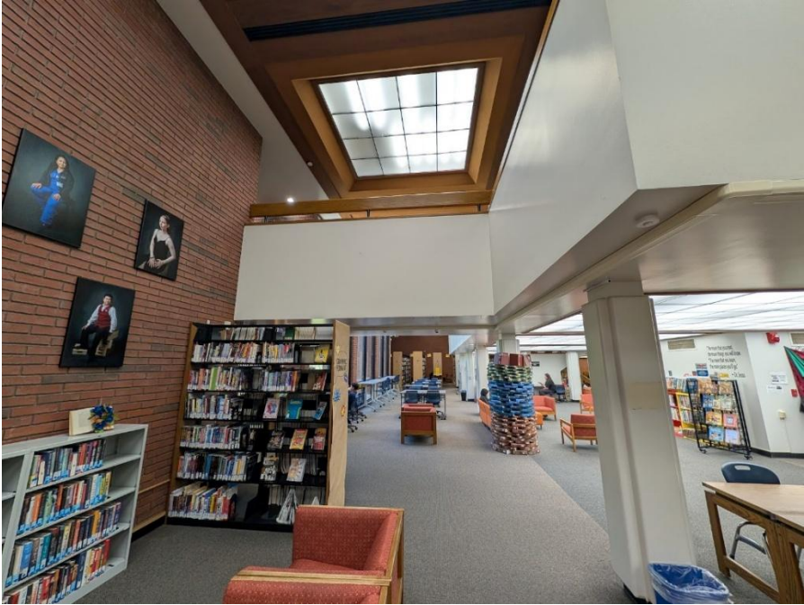
Photo C3 – Mezzanine Columns at Gridline D (Proposed Braced Frame Line)
