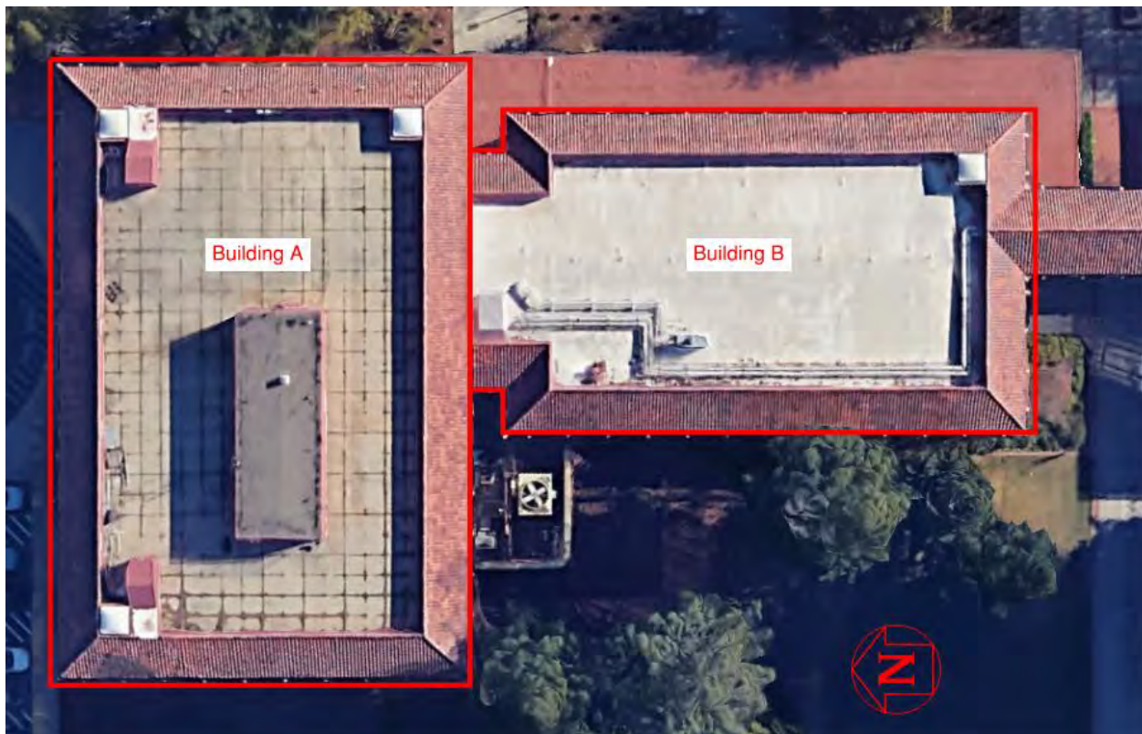
Figure 1 – Rodda Hall Buildings A and B
