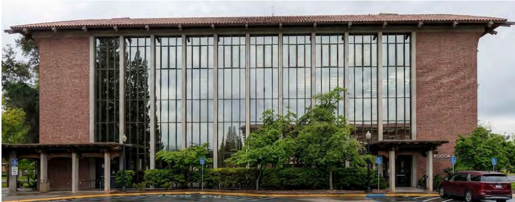
Photo C1 – Rodda Hall North Elevation
