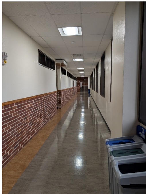
Photo C2 – Rodda Hall Typical Hallway with Window Openings on Right
