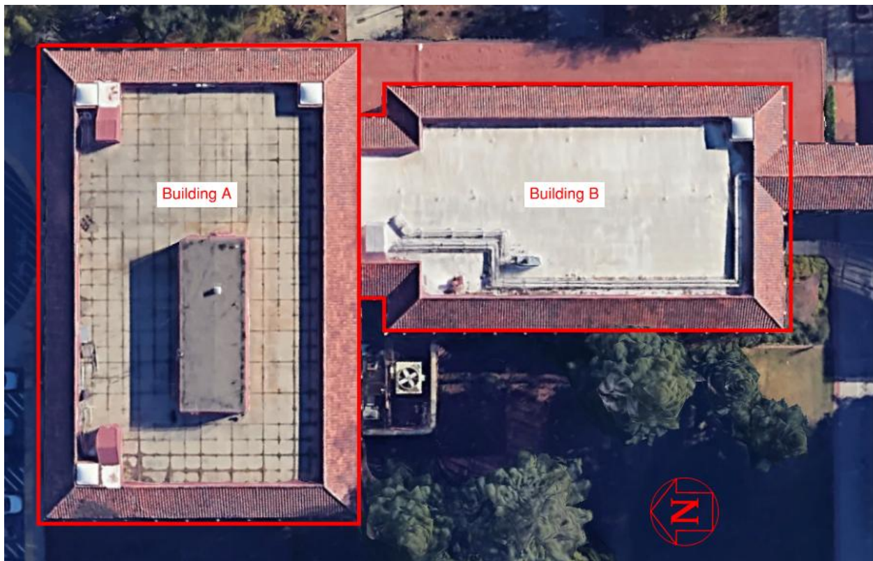
Figure 1 – Rodda Hall Buildings A and B
