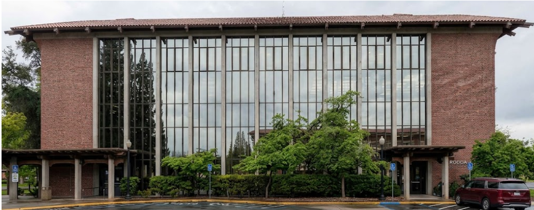
Photo C1 – Rodda Hall North Elevation
