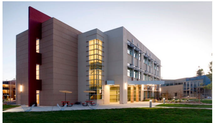
SCC West Sacramento Center
