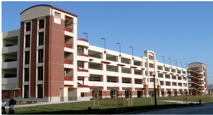
SCC Parking Structure
