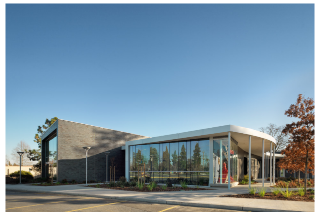
ARC Life Science & Fine Arts Modernization
