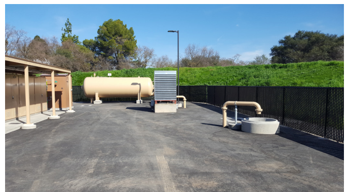
ARC Water Well Replacement
