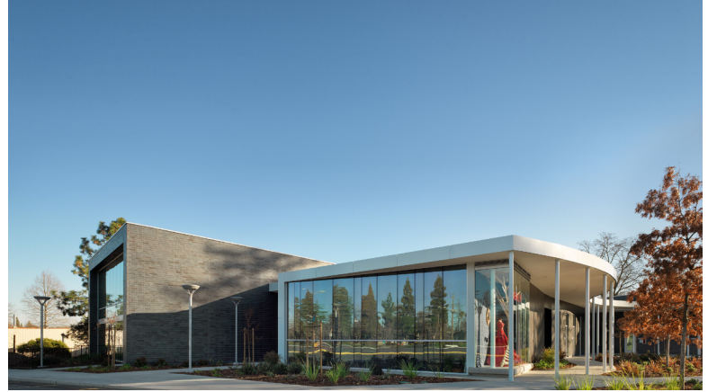
ARC Life Science & Fine Arts Modernization
