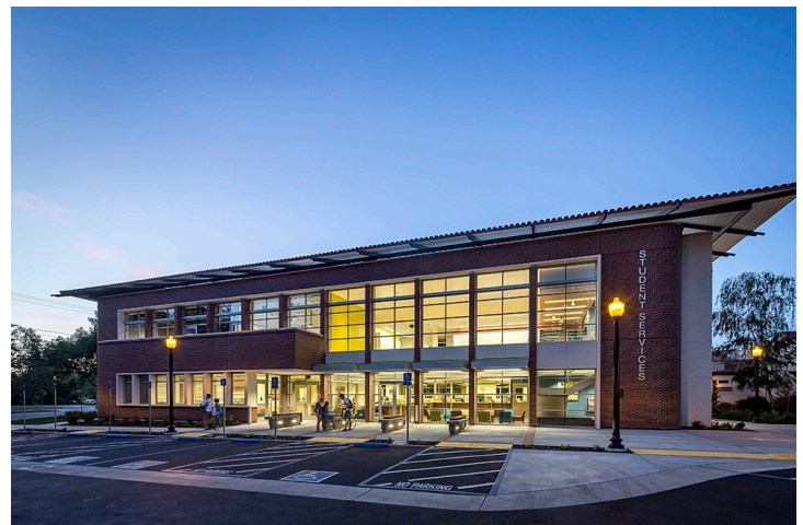
SCC Student Services Modernization and Expansion
