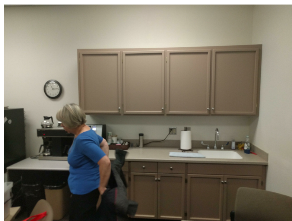
2 COLLEGE CENTER BREAK / WORKROOM: REMOVE (E) COUNTERTOP, CASEWORK, PLUMBING, ETC. CAP PLUMBING BEHIND WALL & FINISH WALL TO MATCH ADJACENT WALL SURFACE
